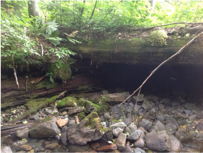
Left Bank Abutment when facing downstream
